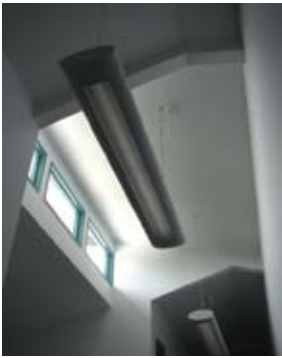
Views of the GAC office complex.
